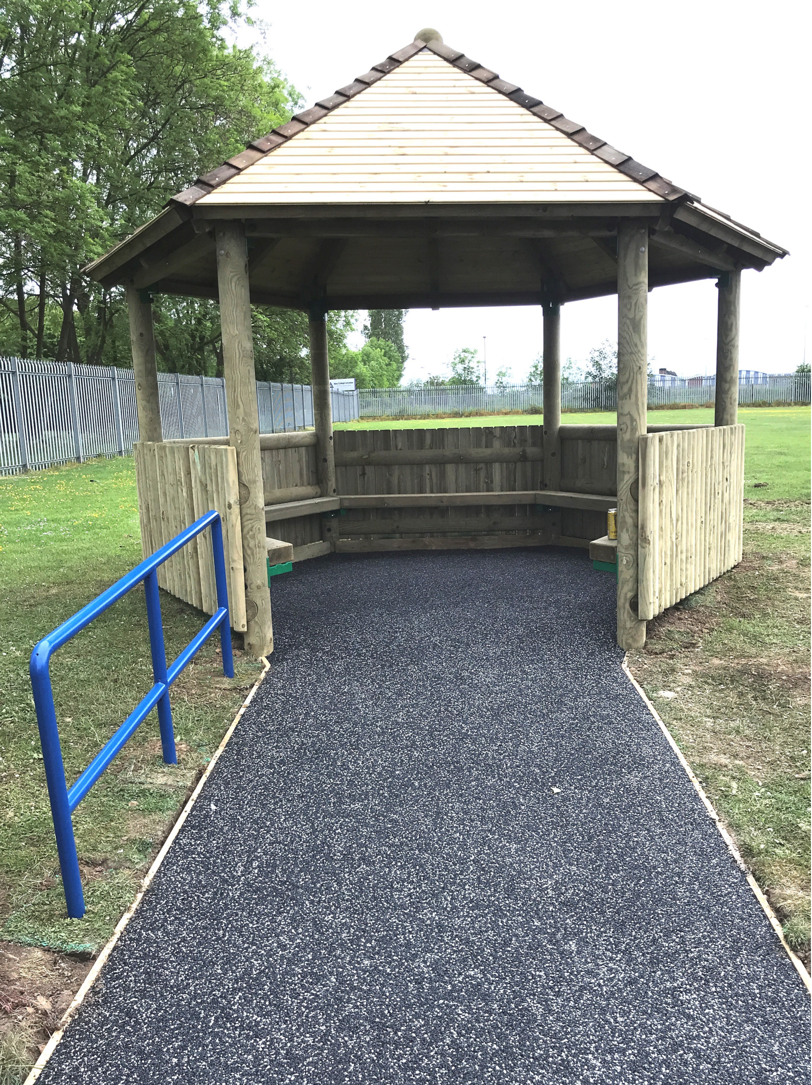
Path and Shelter Base installation using Conipave Silver
